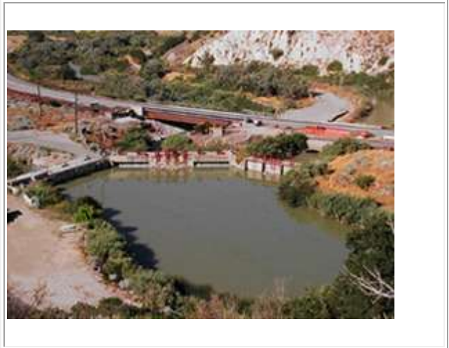
The Turner Dam located at the Jordan Narrows is a major diversion works on the Jordan River.
