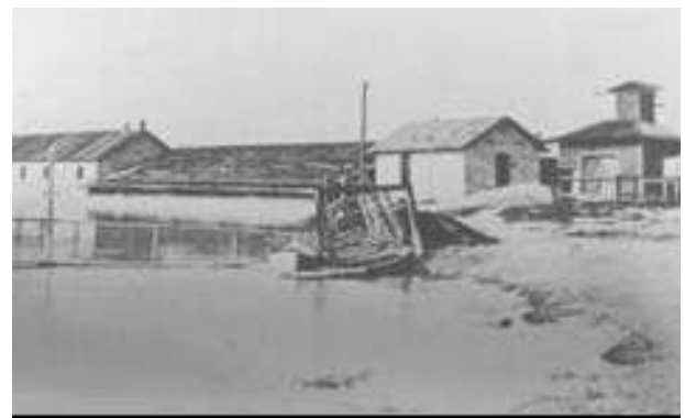
The Utah Lake Pumping Plant, owned by the Associated Canals, is located at the outlet of the lake. In 1907 this was the largest pumping plant in the United States, capable of pumping 700 cfs or 452 mgd.
