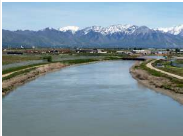
The Surplus Canal near the Salt Lake International Airport is conveying high flows to the Great Salt Lake. Flows have already reached 4,000 cfs.
