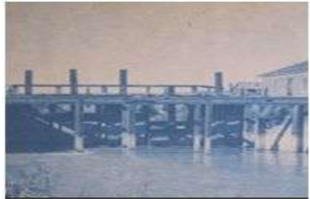
The "Old Dam" located at the Jordan Narrows was built by the County in 1872. Under the same project the County began construction of the Utah and Salt Lake Canal. The dam consisted of timber uprights set in cement, between which planks were inserted to raise water into the East Jordan and Utah and Salt Lake Canals.
