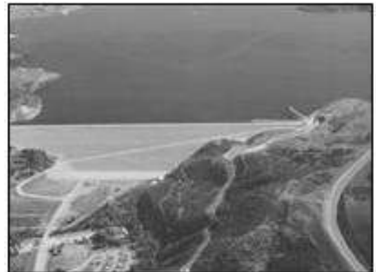
Central Utah Project Jordanelle Dam located northwest of Heber City.
